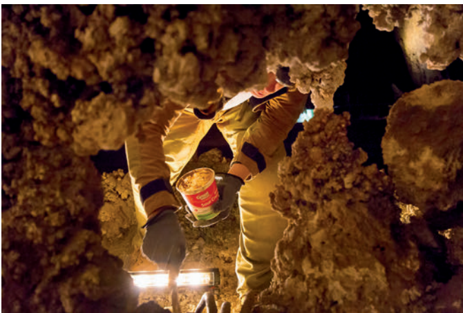
Brushing “slurry” mixture over a cable run. Photo by Evan Hubbard.
