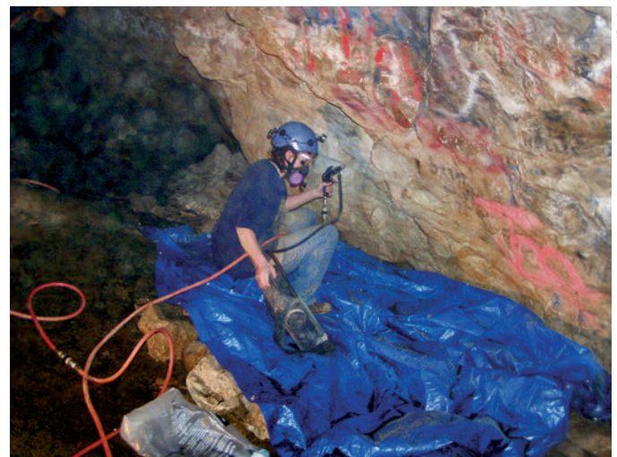
Using the sandblaster to remove paint markings
