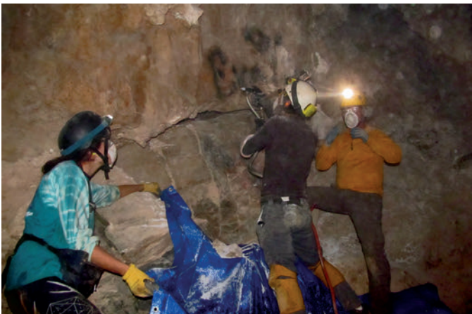
Sandblasting with protective gear and tarps (R. Keeler)
